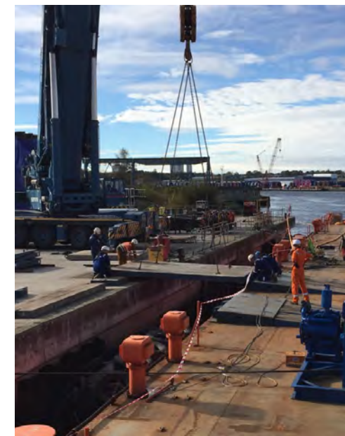
fig. 2 / Linkspan pieces being installed to barge for loadout
