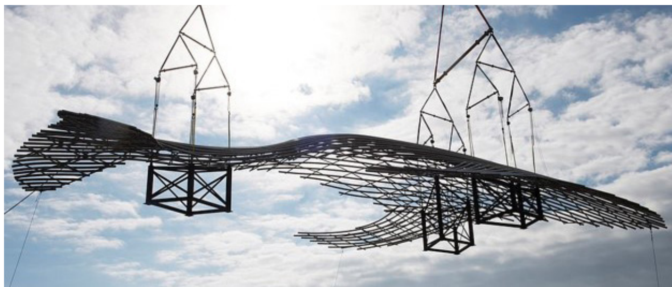
Figure 5: The Tay Whale Supported by the complex 11 beam lift arrangement
