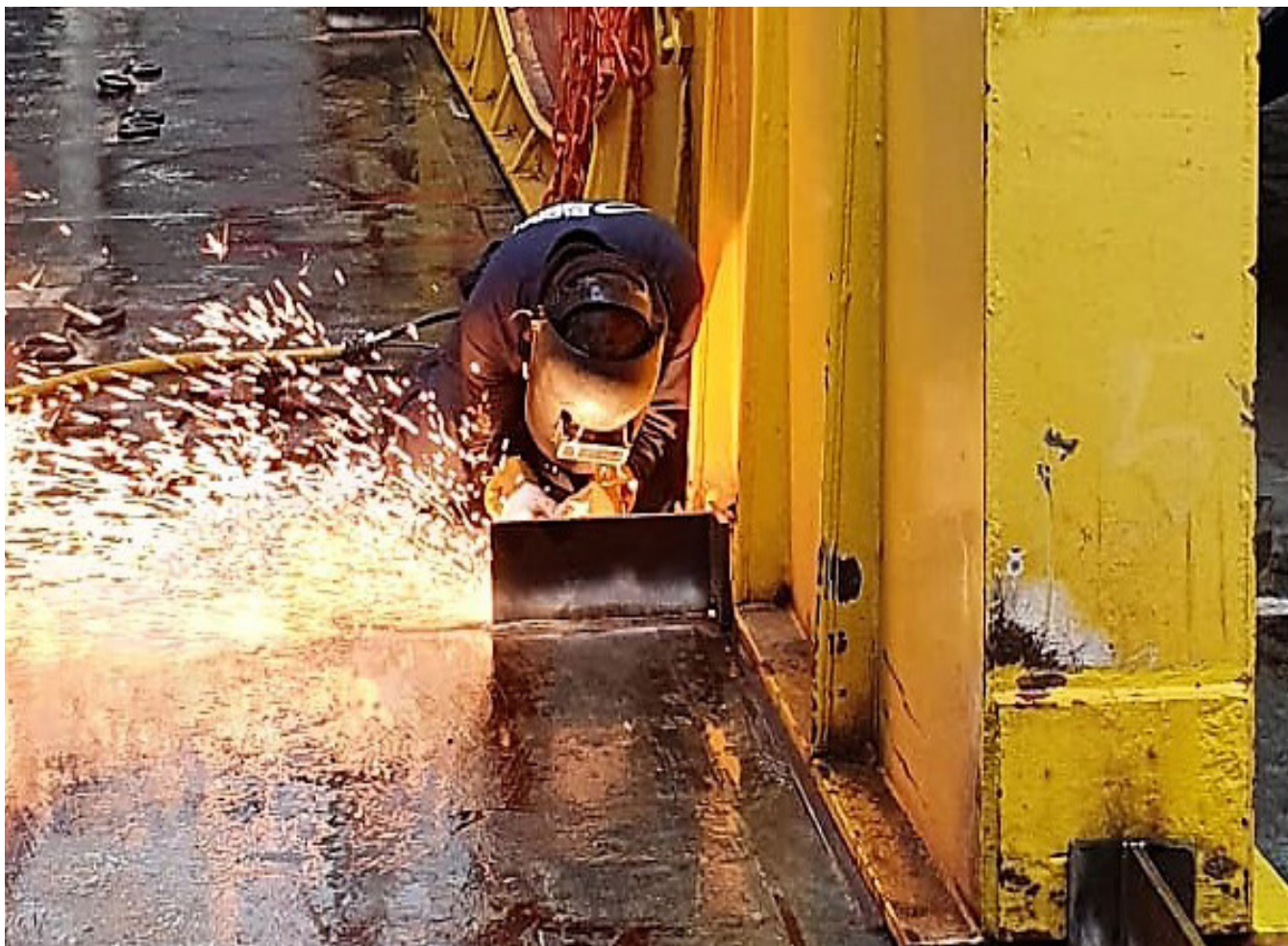
Figure 5: Seafastening removal
