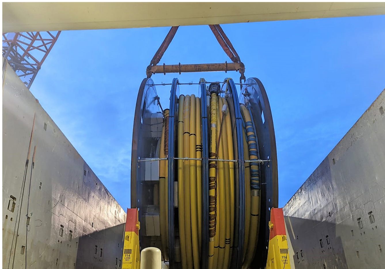
Figure 3: 11.4m reel lifted from vessel hold
